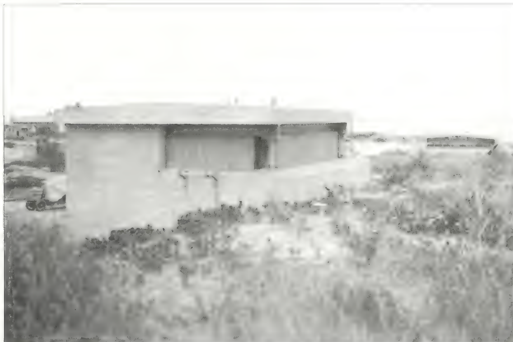
Figure 5.35. Batteries Engle and Peck circa 1920. The battery commander's station for Battery Peck is seen in the foreground. The low concrete structure seen in the background is the coincidence range finder station built into the former gun emplacement of Battery Engle in 1920. Note the low-growing vegetation in this photograph, making possible downrange views and effective operation of the batteries (GATE 7892).
